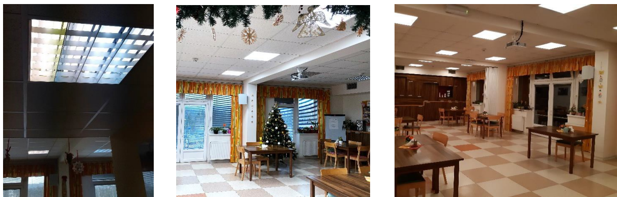
Figure 4: Dining room lighting: A – detail of an original fixture with reflective grates; B – comparison between the original (right) and new (left) lighting in the day mode; C – new lighting in the evening mode.
