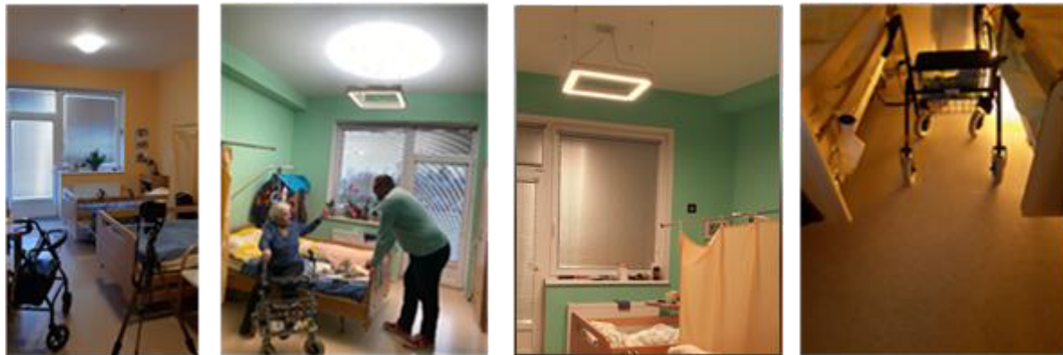
Figure 2: Lighting in the clients' rooms. The original light (A) was replaced with a biodynamic lighting system with variable spectral composition, light emission characteristics and light intensity matching the day/evening time (B, C). Orientation glow lights were installed in the rooms to facilitate clients' movements during the night (D).
