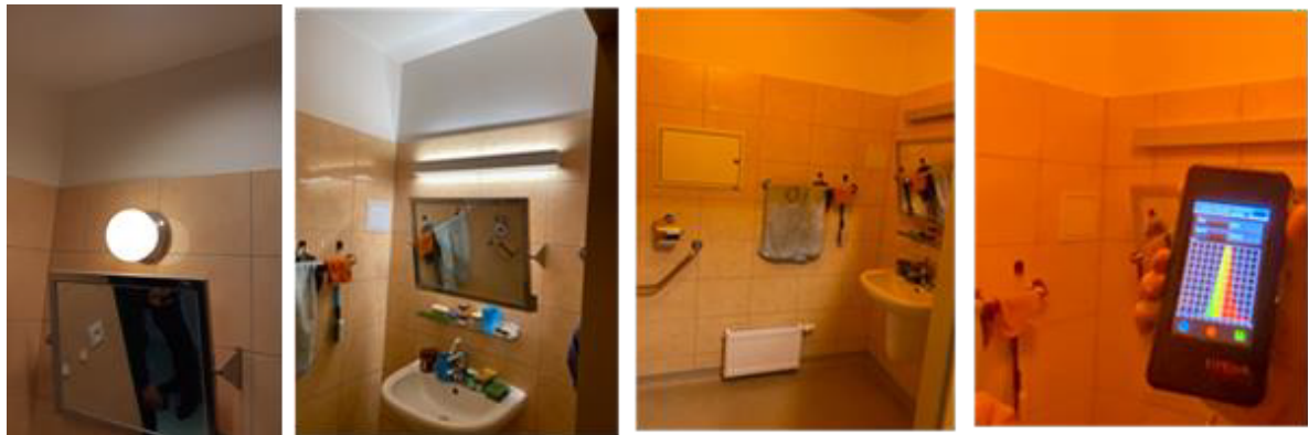
Figure 3: Bathroom lighting. A – The original lighting was strengthened and light distribution was changed (B). The system was completed with a night mode (C, D).
