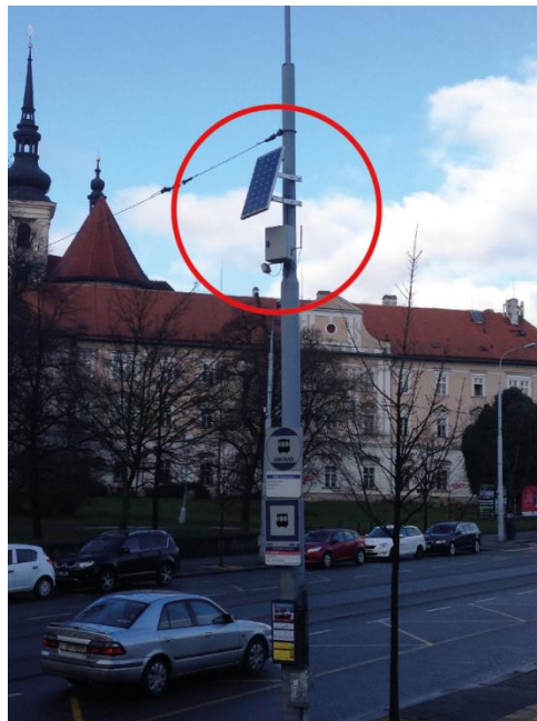
Master SOLAR - CM 1212 (60 W PV panel, 33Ah aku)
